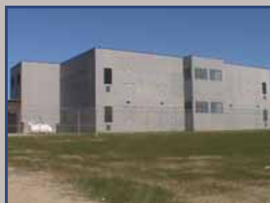
J. Reuben Long Detention Center Bed Tower Conway, SC
