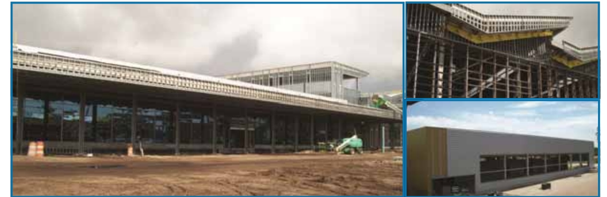
Myrtle Beach International Airport Terminal Capacity Enhancement Project
